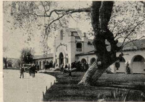
ENTRANCE ACUA CALIENTE HOTEL
