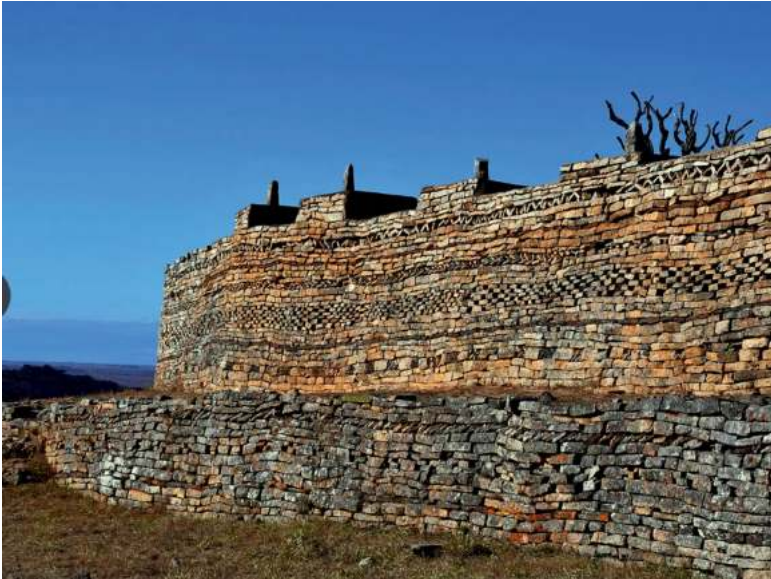
Detail of a wall in Khami. Image: ICCROM Archive.
