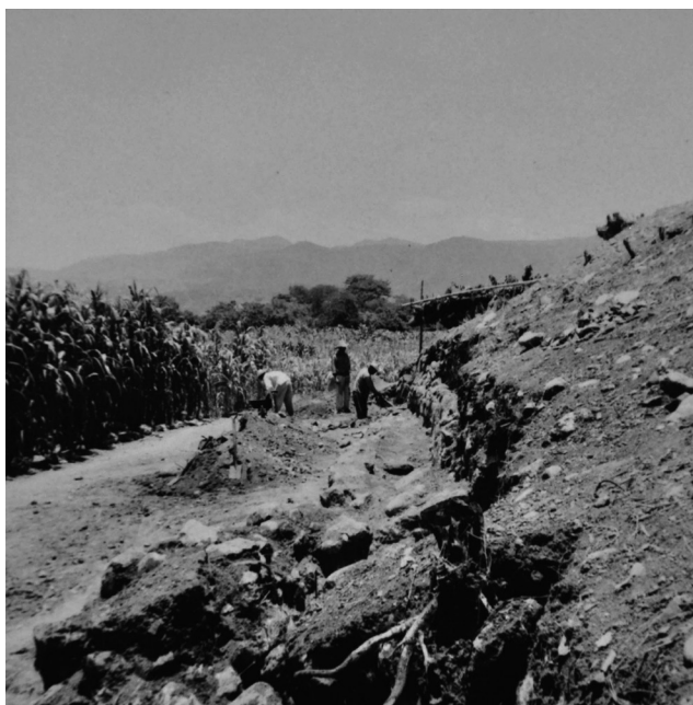
West End, Beginning of Excavations, Looking North.
