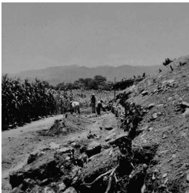
West End, Beginning of Excavations, Looking North.
