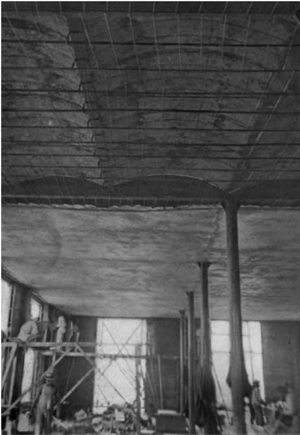
Figura 10. Fire proof ceiling, Havana Cigar Factory, Taken during construction, showing part plastered and balance with reinforcing metal work. Work designed, furnished and erected by Milliken Brothers. Milliken Brothers, Nueva York, 1905, p. 121.
