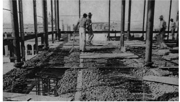
Figura 9. Floor arching, Havana Cigar Factory, taken during construction, showing method of constructing floor arches with reinforcing metal and flooring in concrete. Work designed, furnished and erected by Milliken Brothers. Milliken Brothers, Nueva York, 1905, p. 120.
