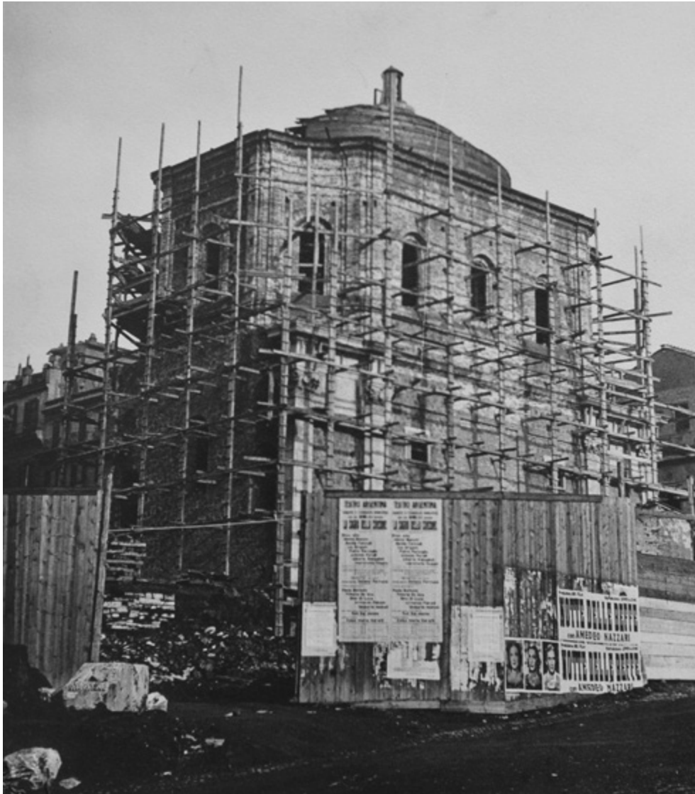
Figure 5. Reconstruction of Santa Rita de Cascia (originally built by Carlo Fontana, in 1665), Rome, moved from the foot of Ara Coeli to the vicinity of Teatro Marcelo. Image: Gustavo Giovannoni, 1928.
