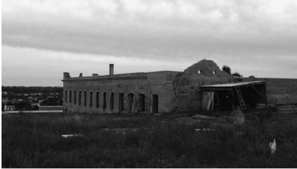
Figure 7. Infirmary of Jaguarão where the preserved ruin and part of the reinforced concrete curtain can be perceived. Image by the author.
