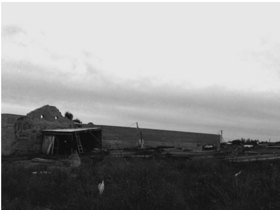
Figure 6. Infirmary of Jaguarão where the extended drapes of reinforced concrete came be seen. Image by the author.
