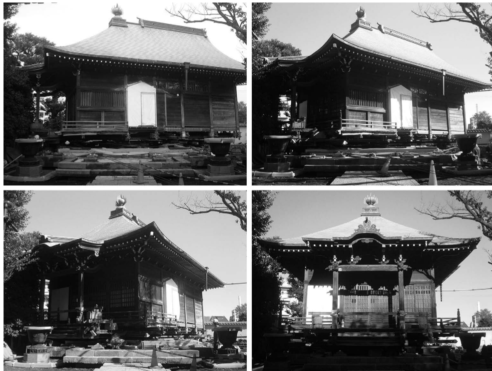
FIGURE 2. MOVEMENT AND ROTATION OF THE TEMPLE YUTENJI, MEGURO, TOKYO, 2014. Image: José Miguel Silva.
