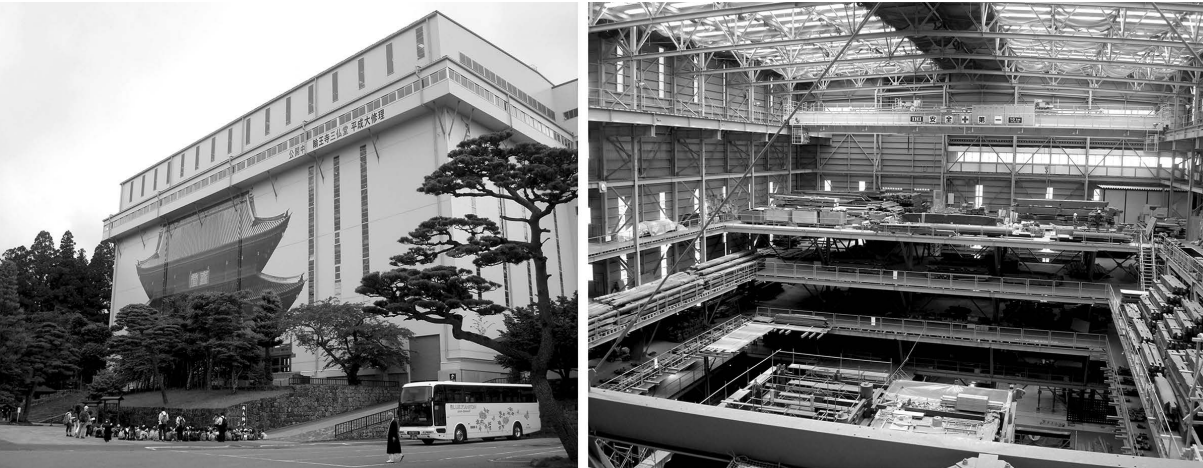
FIGURE 3. THE RINNŌJI TEMPLE, NIKKO, TOTALLY DISMANTLED FOR ITS RESTORATION, 2014. Image: José Miguel Silva.
