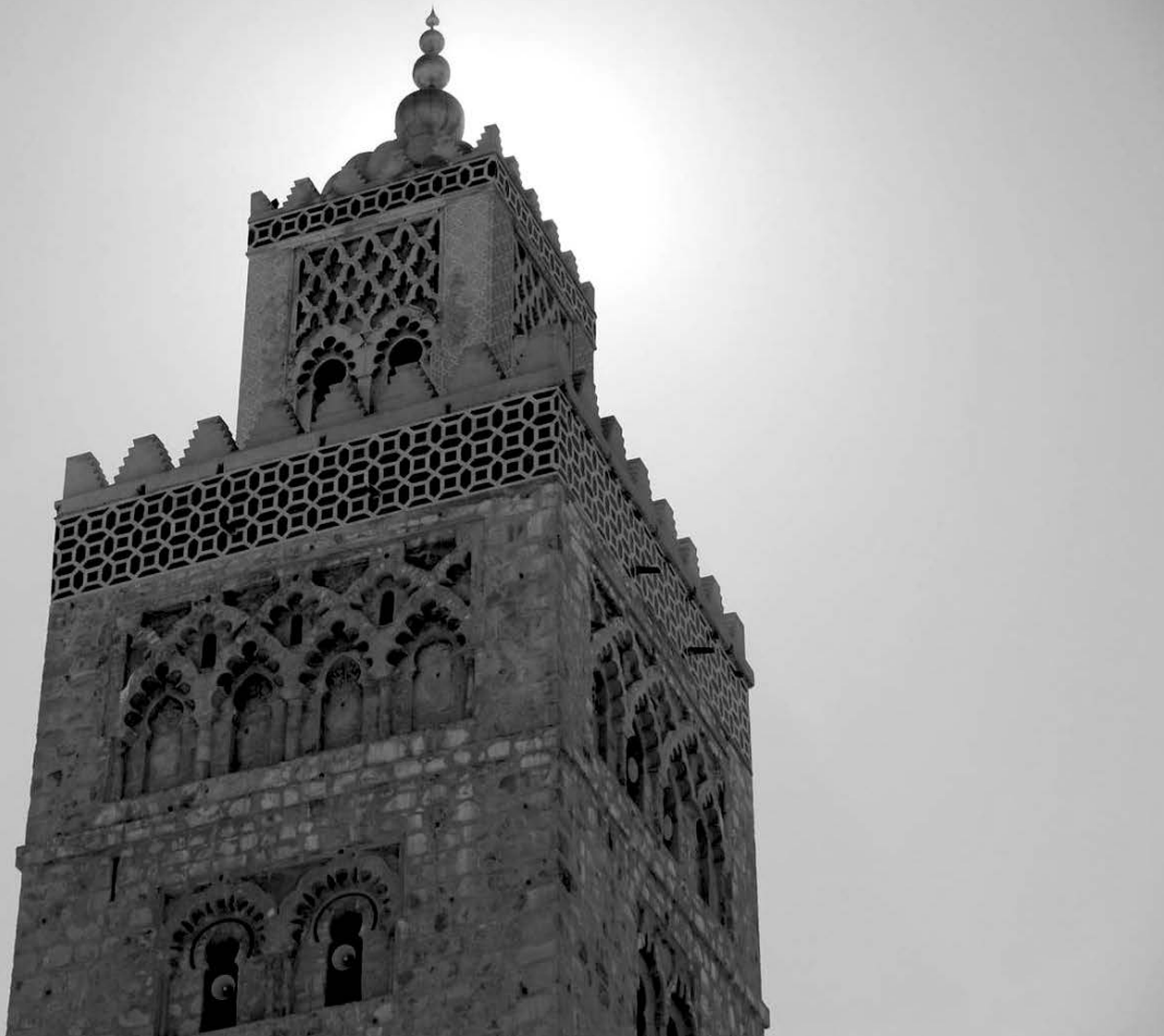
FIGURE 10. MINARET OF THE ALMOHAD MOSQUE OF THE KOUTOUBIA OF MARRAKECH. Condition after the restoration of the tile in its upper area using traditional techniques. Image: Pablo Herrero Lombardia.
