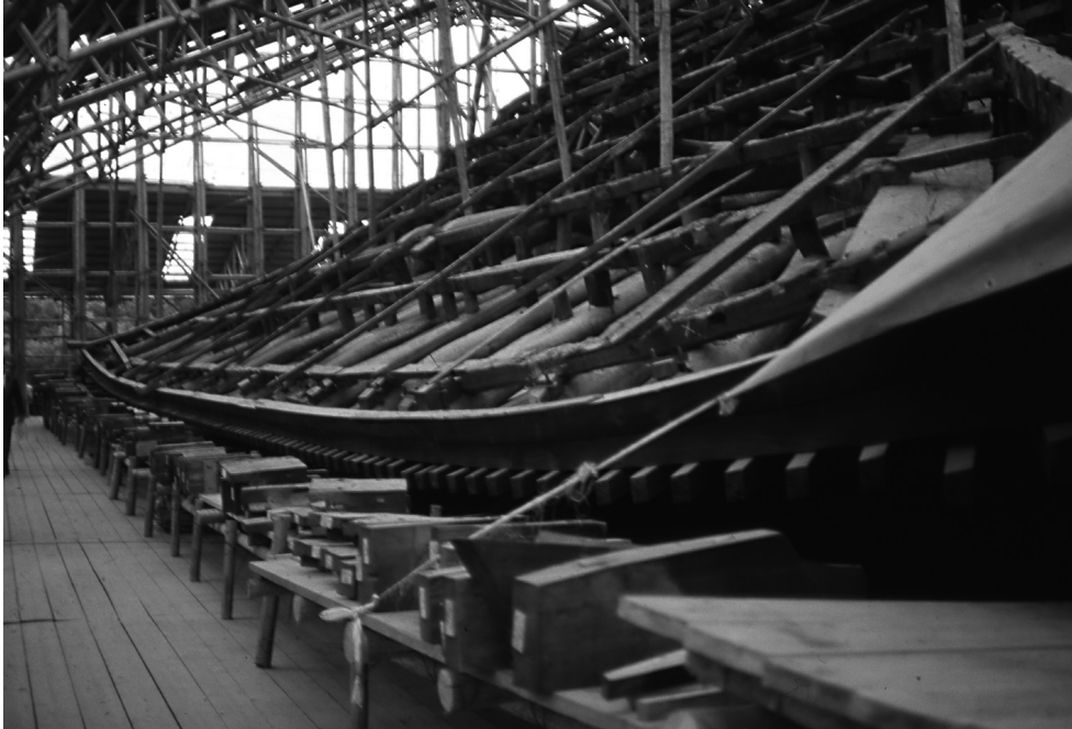
RESTORATION OF WOODEN TEMPLE. Fearing that World Heritage nominations would be judged within Eurocentric frameworks, the Japanese were also concerned that existing widespread conservation practices –such as the top-to-bottom periodic dismantling and reassembly of significant religious structures– would also be misunderstood by Western evaluators. Image: Herb Stovel, 1993, ©ICCROM.
