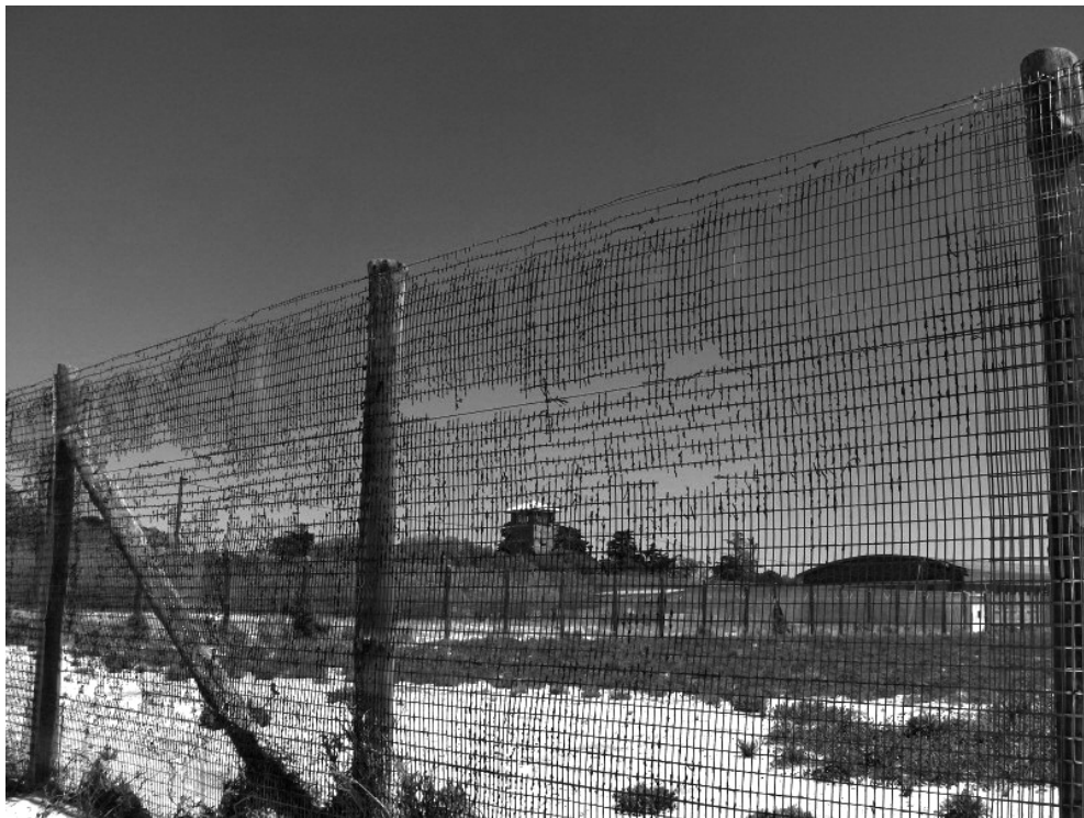
MAXIMUM SECURITY PRISON. Fence disposed during maintenance works. Image: ©Pascall Taruvinga, 2019.
