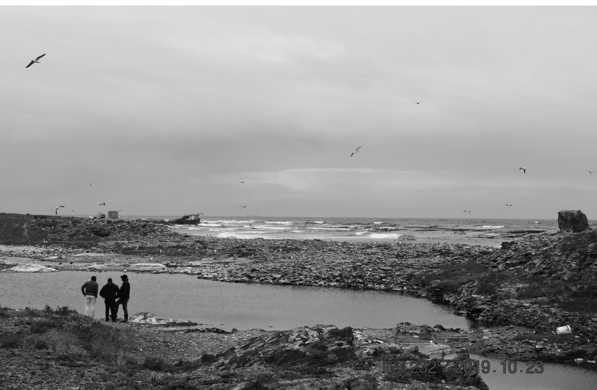
BLUE STONE QUARRY SITE. Progressive collapse of the wall. Image: ©Pascall Taruvinga, 2019.
