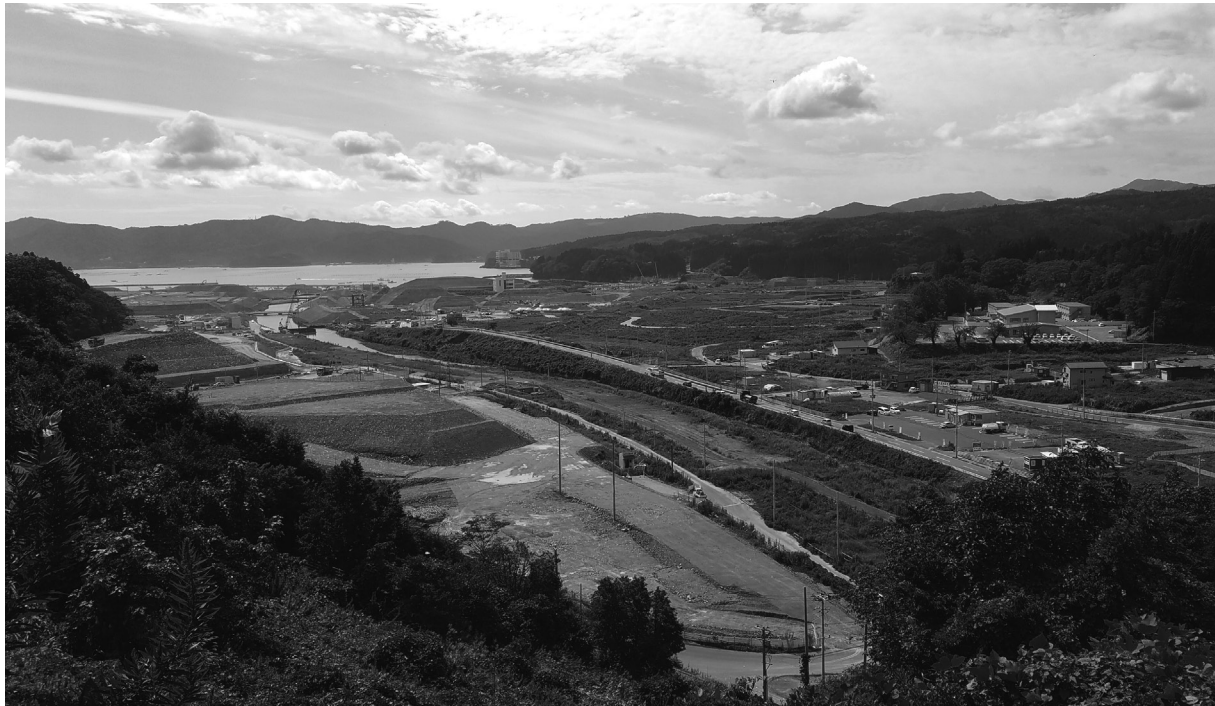
TRADITIONAL FISHING VILLAGE OF SHIZUGAWA IN MINAMISANRIKUCHO. It was nearly wiped out due to 2011 Great East Japan Tsunami. Image: Rohit Jigyasu.
