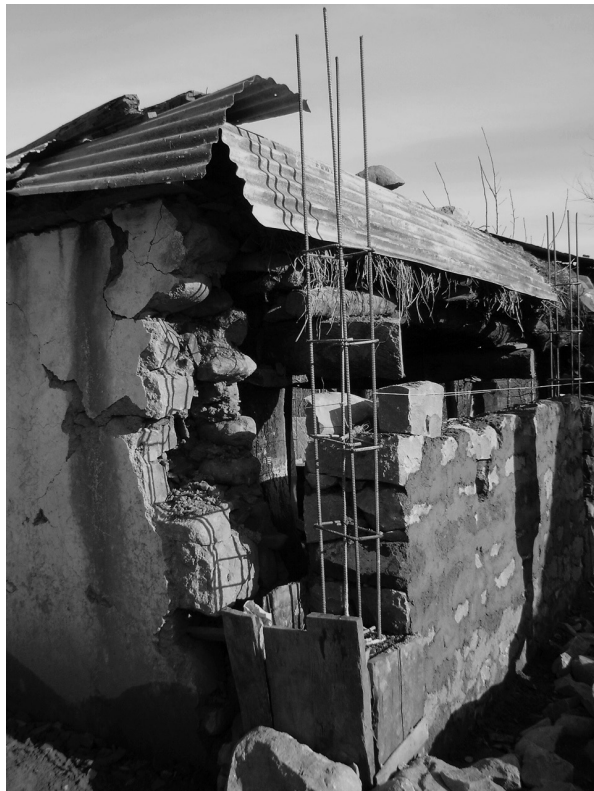
MARATHWADA, INDIA. Local masons carry out unsafe construction practices using new materials and technology because of lack of appropriate knowledge and unaffordability. Image: Rohit Jigyasu.
