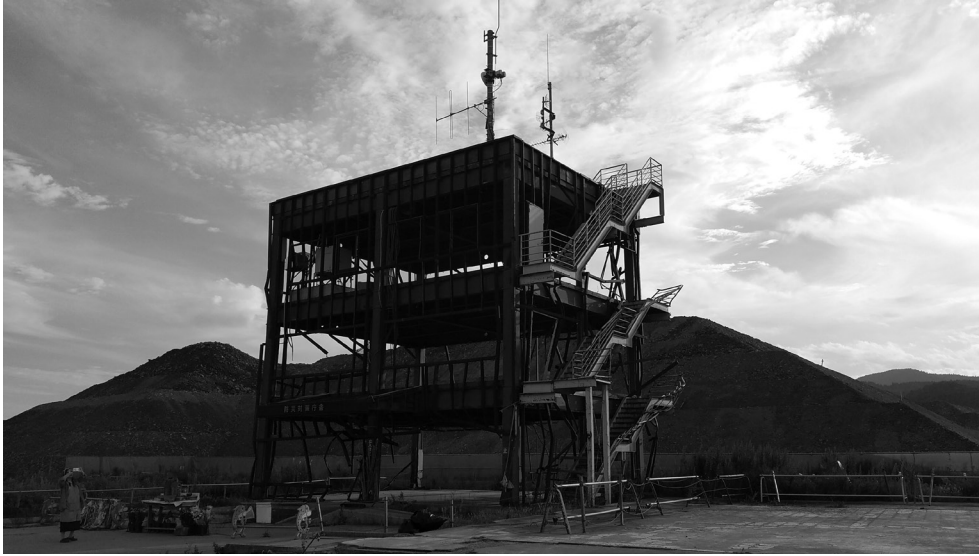
SHIZUGAWA, JAPAN. The skeleton of disaster prevention centre located in the middle of Shizugawa town following massive damage due to the 2011 Great East Japan Tsunami has become a popular place for visitors. Image: Rohit Jigyasu.
