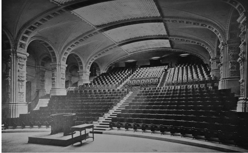
FIGURE 5. VAULT OF THE AMPHITHEATRE OF THE ENP, ANNEX, 1910. Image: Chávez, 1911.
