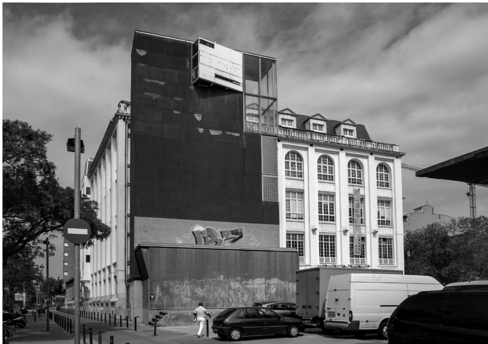
FIGURE 2. CENTRE CIVIC CAN FELIPA. BARCELONA. BEFORE: FÀBRICA TEXTIL CATEX, BENET PUIG I ROSSINYOL, 1856. Intervention by Josep Lluís Mateo i Martínez, 1984-1991. Image: Carlos Colás.
