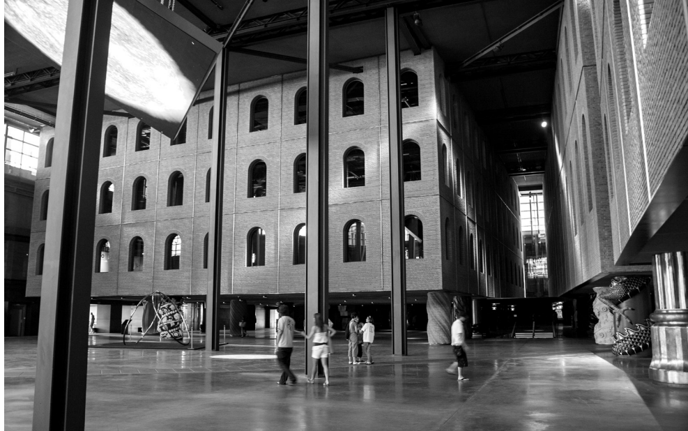
FIGURE 4. AZKUNA ZENTROAZ. BILBAO. BEFORE: ALHÓNDIGA, RICARDO BASTIDA, 1905-1909. Intervention by Philippe Starck, 2001-2010. Image: Carlos Colás.
