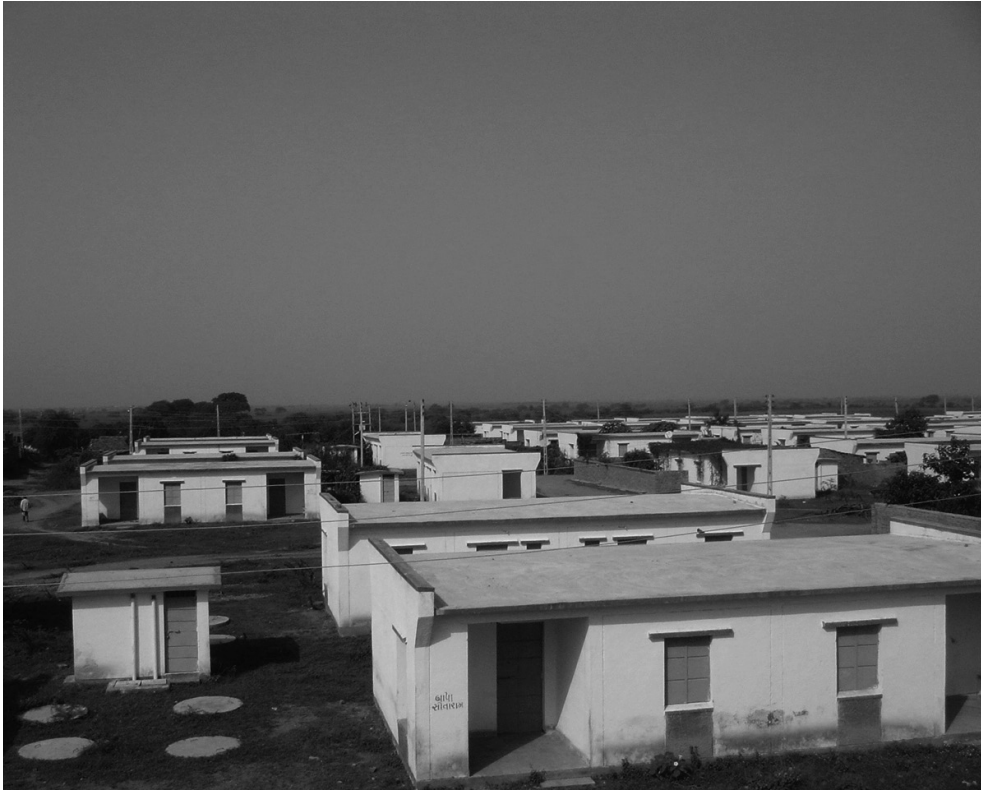
MARATHWADA, INDIA. The house designs and the layout of villages reconstructed after the 1993 Marathwada earthquake in India had no link with traditional architecture and planning. As a result, many of these villages were not occupied by the beneficiaries, who preferred to reconstruct their traditional shelter. Image: Rohit Jigyasu.
