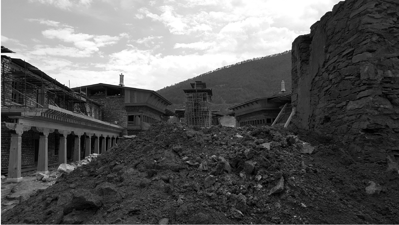
WANGDUAPHODRANG ZHONG, BHUTAN. Reconstruction following a devastating fire in 2012 through engagement of local craftsmen. Image: Rohit Jigyasu.
