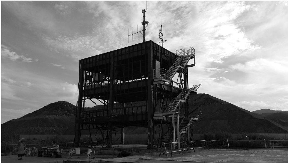
SHIZUGAWA, JAPAN. The skeleton of disaster prevention centre located in the middle of Shizugawa town following massive damage due to the 2011 Great East Japan Tsunami has become a popular place for visitors. Image: Rohit Jigyasu.
