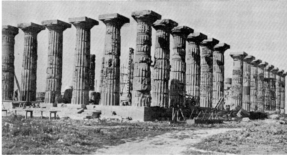
FIGURE 3. RESTORATION OF THE TEMPLE E IN SELINUNTE BY NAPOLEONE GANDOLFO. Survey and views before and after intervention. Image: Dezzi Bardeschi e Sanpaolesi (1964: np).
