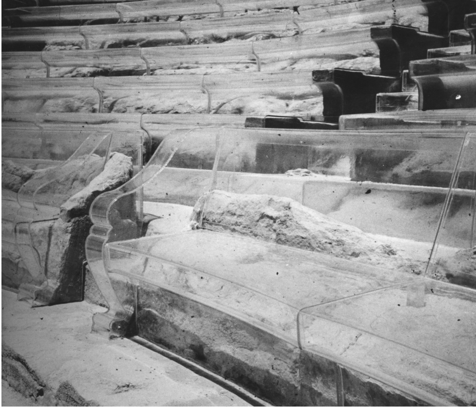
FIGURE 1. HERACLEA MINOA HELLENISTIC THEATRE'S CAVEA. Restoration of the cavea using synthetic resin by Franco Minissi. Image: ©ICCROM.
