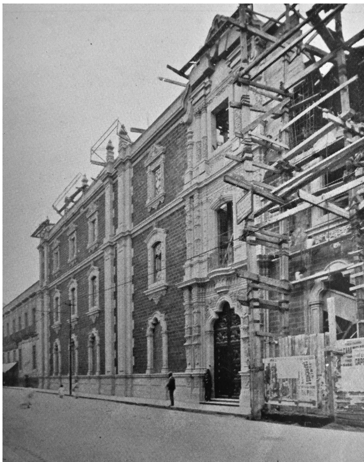
FIGURE 4. FAÇADE OF THE ANNEX IN 1910. Image: Chávez, 1911.
