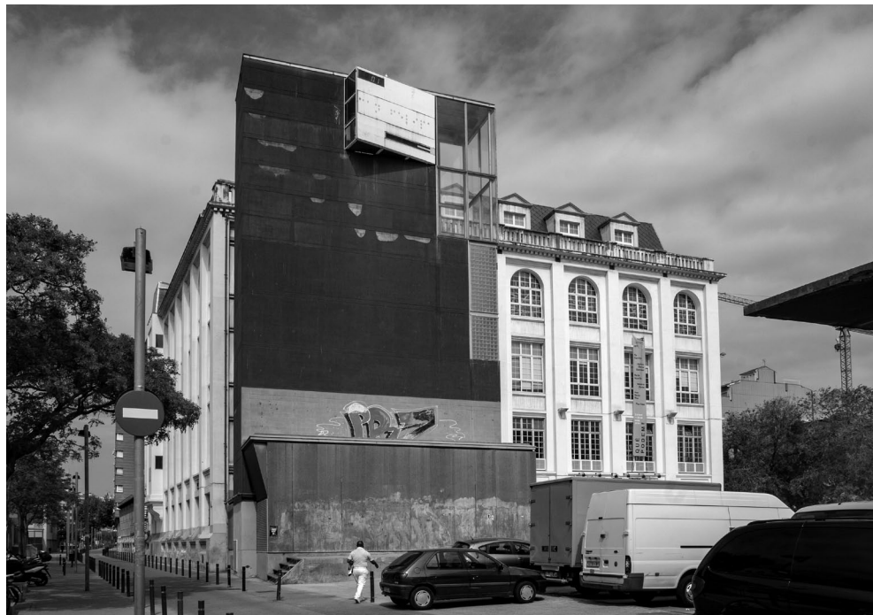
FIGURE 2. CENTRE CIVIC CAN FELIPA. BARCELONA. BEFORE: FÀBRICA TEXTIL CATEX, BENET PUIG I ROSSINYOL, 1856. Intervention by Josep Lluís Mateo i Martínez, 1984-1991. Image: Carlos Colás.
