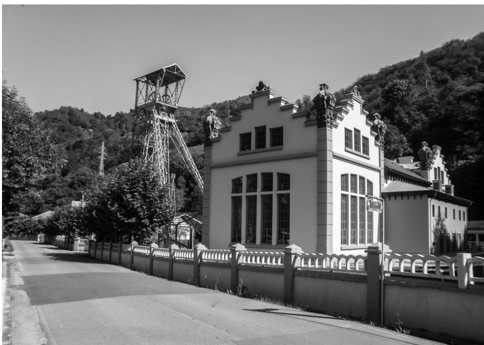
FIGURE 3. ECOMUSEUM OF THE VALLEY OF SAMUÑO. POZO DE SAN LUIS, CIAÑO (LANGREO, ASTURIAS). BEFORE: IT WAS ACTIVE FROM 1928-1969. Definitive closure in 2002. Listed as a site of Cultural interest in 2013. Image: Carlos Colás.
