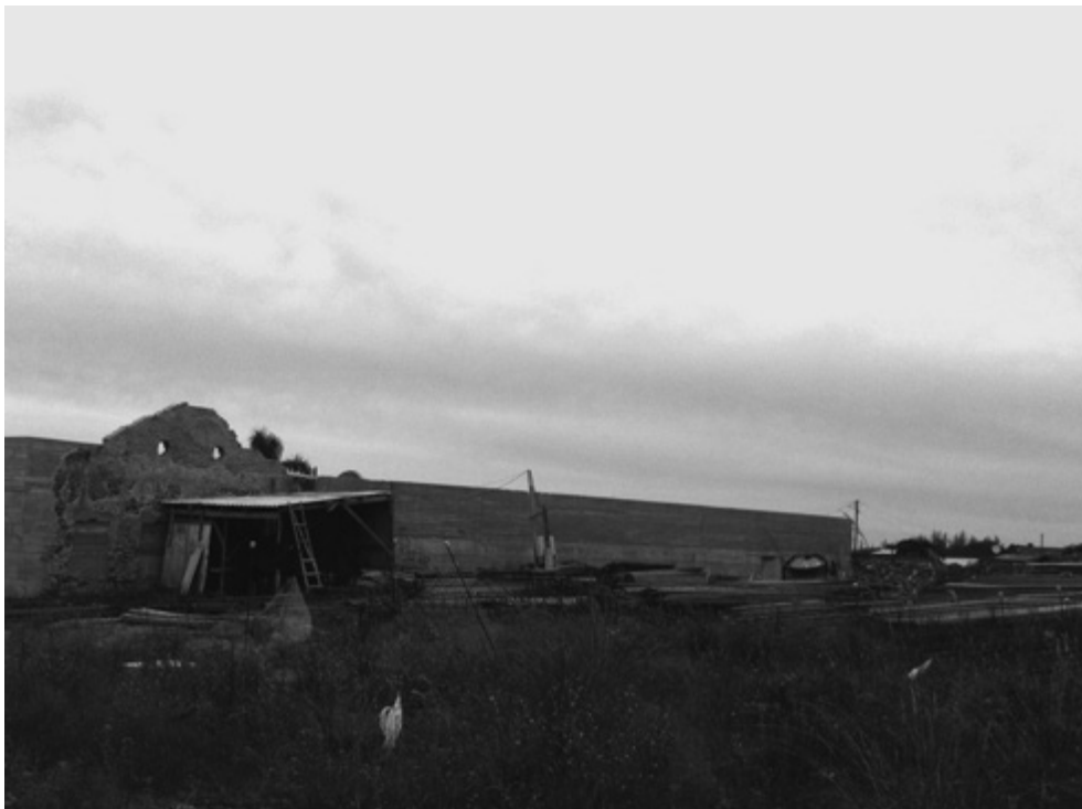
Figure 6. Infirmary of Jaguarão where the extended drapes of reinforced concrete came be seen. Image by the author.
