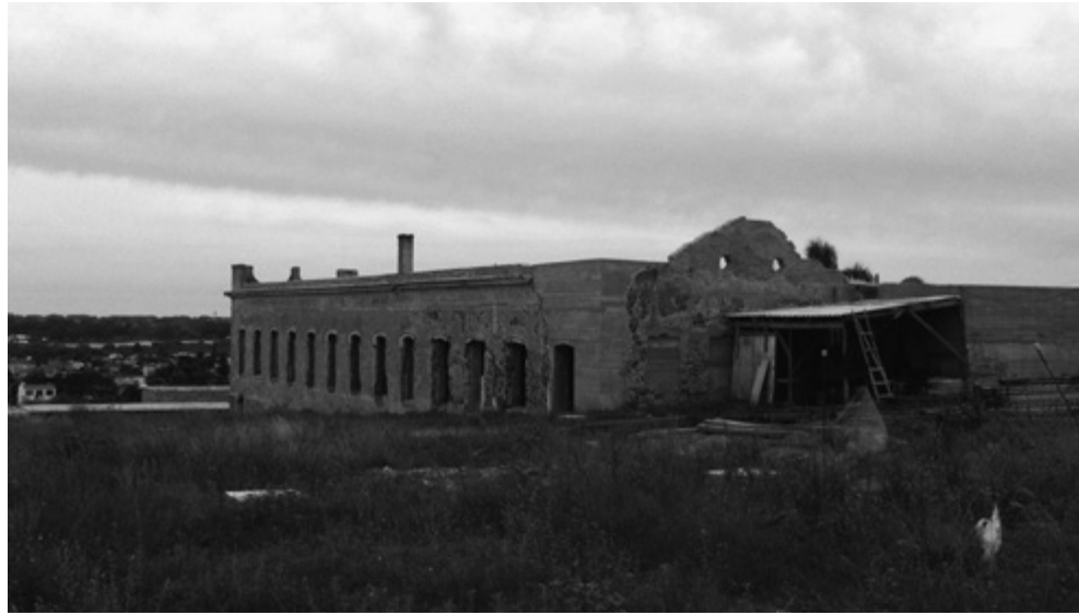
Figure 7. Infirmary of Jaguarão where the preserved ruin and part of the reinforced concrete curtain can be perceived. Image by the author.
