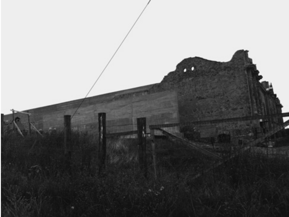
Figure 5. Infirmary of Jaguarão where the intervention with reinforced concrete can be seen. Image by the author.
