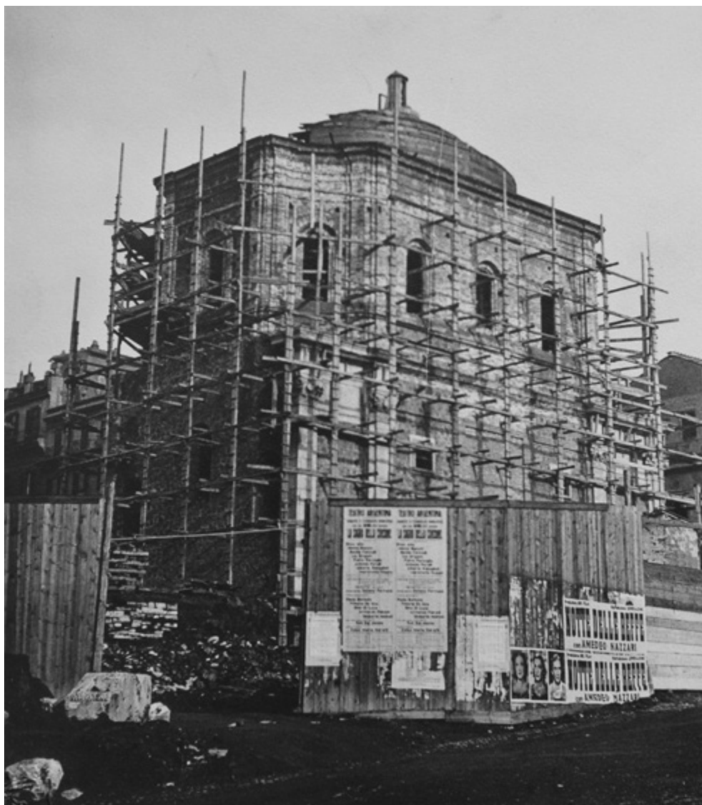
Figure 5. Reconstruction of Santa Rita de Casia (originally built by Carlo Fontana, in 1665), Rome, moved from the foot of Ara Coeli to the vicinity of Teatro Marcelo. Image: Gustavo Giovannoni, 1928.
