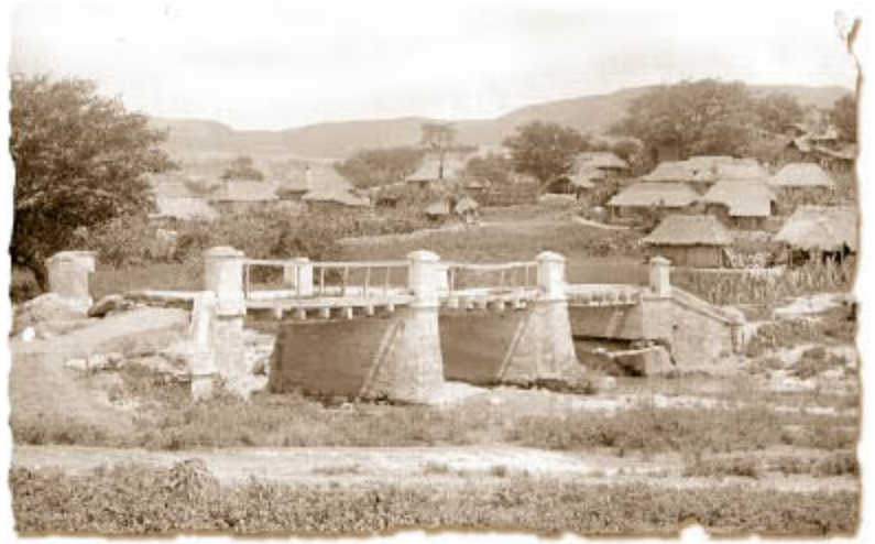
Puente en Chilpancingo que muestra daños en uno de sus soportes, 2 de enero de 1910. © Wicks, S. Robert & Harrison H. Roland, Buried Cities, Forgotten Gods. William Niven's life of discovery and revolution in Mexico and the American Southwest , Texas Tech University Press, 1999.
