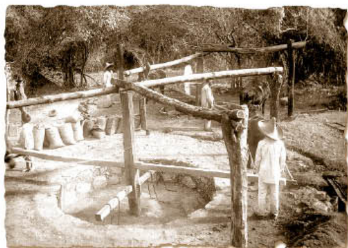
Instalación para trituration de grava, con tracción animal. © Wicks, S. Robert & Harrison H. Roland, Buried Cities, Forgotten Gods. William Niven's life of discovery and revolution in Mexico and the American Southwest , Texas Tech University Press, 1999.
