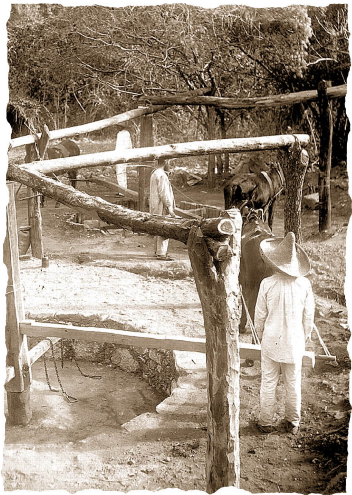
Detalle: Instalación para trituración de grava, con tracción animal. © Wicks, S. Robert & Harrison H. Roland, Buried Cities, Forgotten Gods. William Niven's life of discovery and revolution in Mexico and the American Southwest , Texas Tech University Press, 1999.
