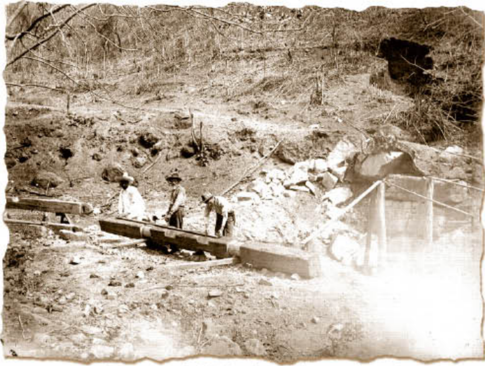
Foto 5: Construcción de un eje para rueda hidráulica. Placeres del Oro. © Wicks, S. Robert & Harrison H. Roland, Buried Cities, Forgotten Gods. William Niven's life of discovery and revolution in Mexico and the American Southwest , Texas Tech University Press, 1999.
