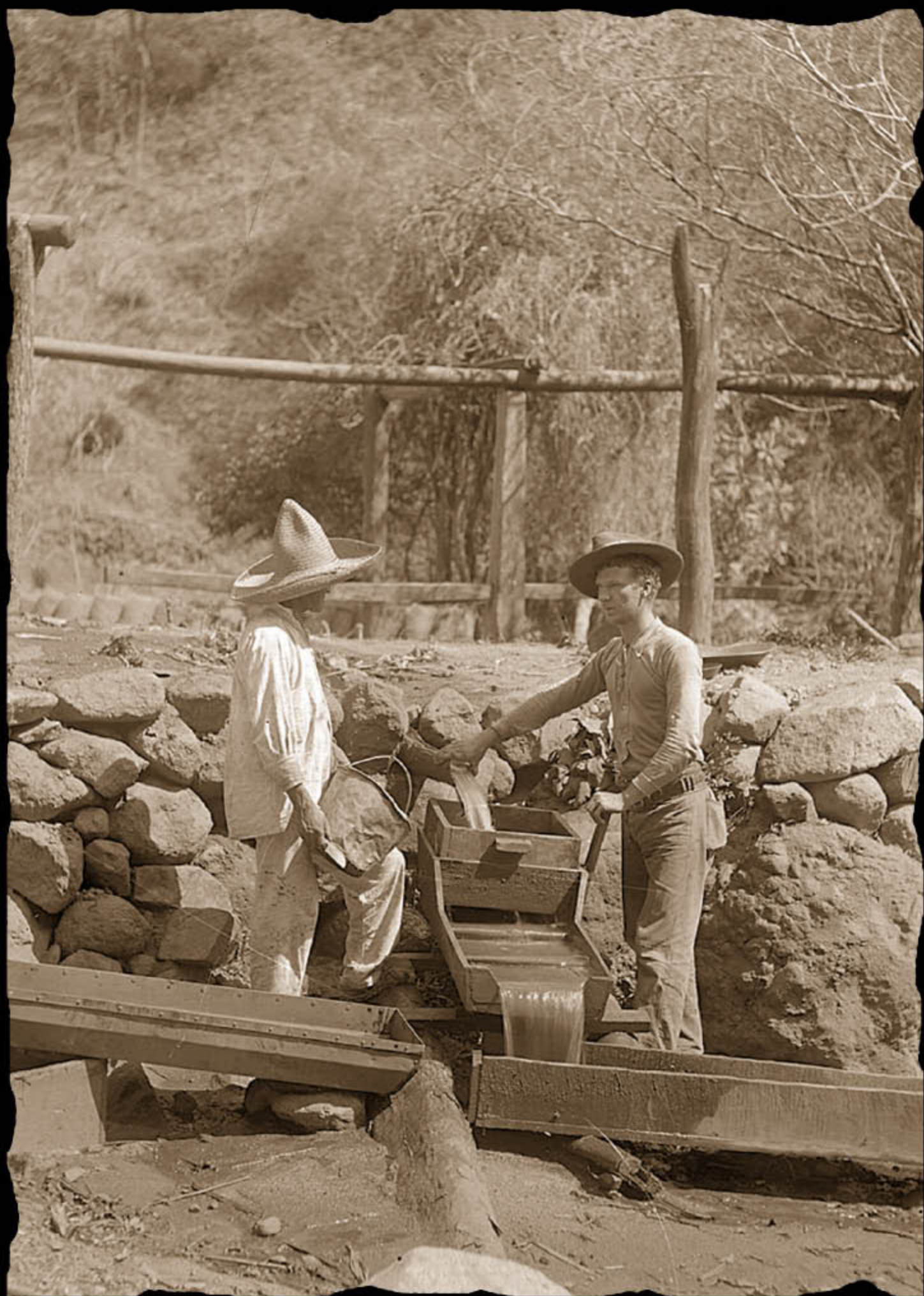
Detalle: Cajonera y contracajonera para el lavado de oro. Placeres del Oro. © Wicks, S. Robert & Harrison H. Roland, Buried Cities, Forgotten Gods. William Niven's life of discovery and revolution in Mexico and the American Southwest , Texas Tech University Press, 1999.
