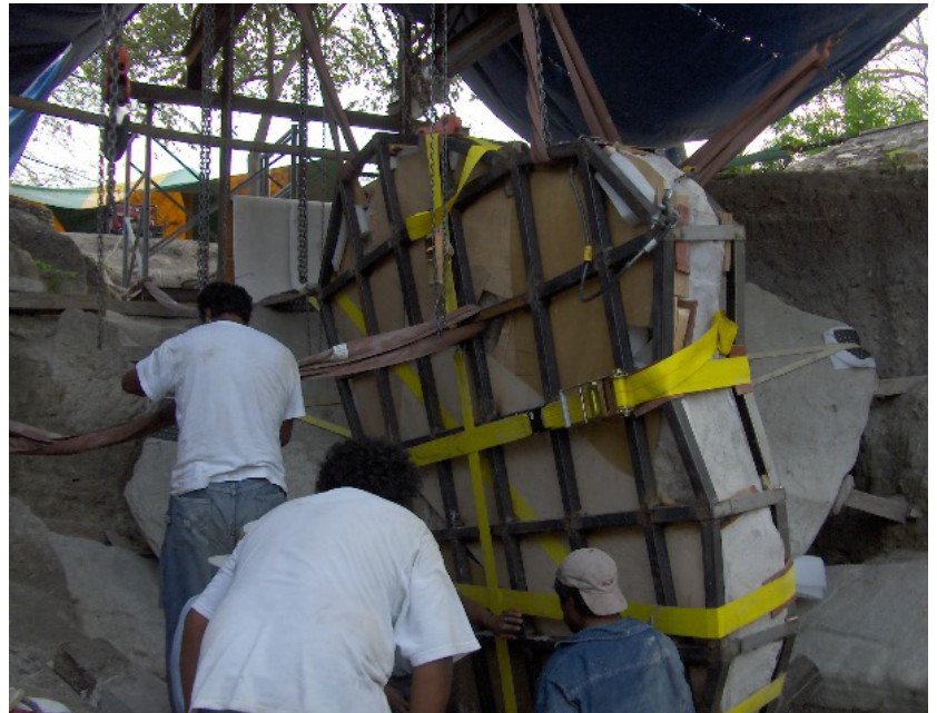
FIGURE 13. Raising of the Venus monolith in the archaeological zone of Tamtoc, San Luis Potosi, Mexico (Source: Dossier of Professor Sergio Montero; ENCRYM-INAH, 2006; courtesy: Iker Montero).
