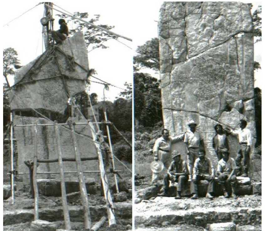
FIGURE 11. Sketch of the process of lifting and reassembling of the fragments of Stele 1 in the archaeological zone of Bonampak, Chiapas, Mexico by Sergio Arturo Montero Alarcón, and images of the restoration of this Stele. (Source: Montero, 1983, p. 72; Dossier of Professor Sergio Montero, ENCRYM-INAH, 1977; courtesy: Iker Montero).
