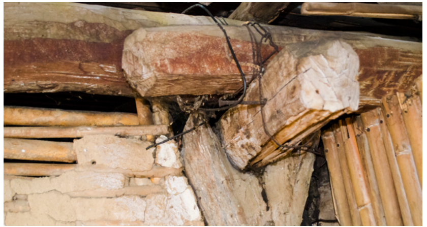
FIGURE 5. Detail of floor slabs underpinning the columns of the vertical structure and wire ties (Photograph: Antonio Flores, 2016).
