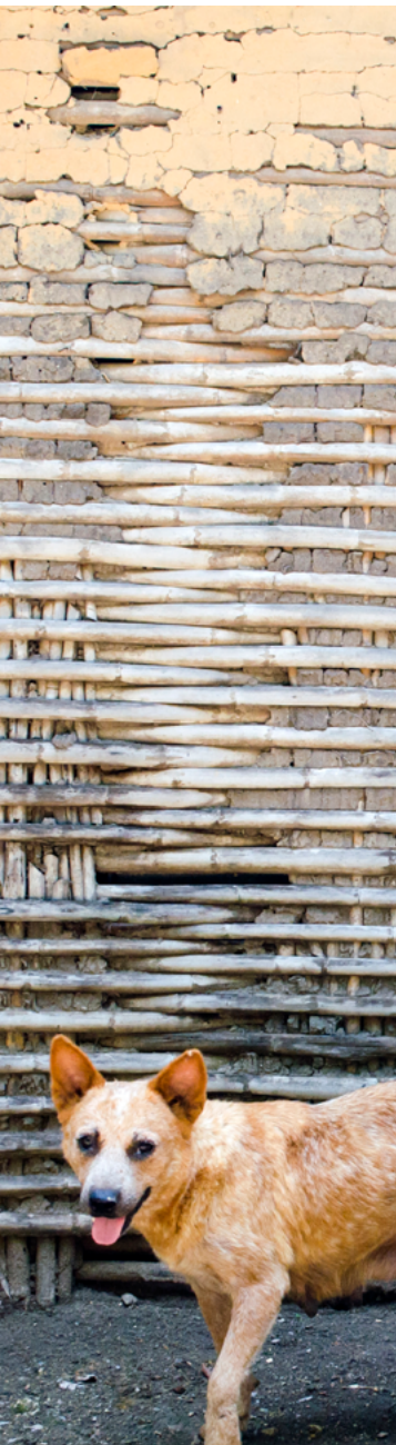
FIGURE 7. Pajarete house located in the community of Pueblo Nuevo displaying the walls of otate and the presence and absence of earth as a finish (Photo: Antonio Flores, 2016).
