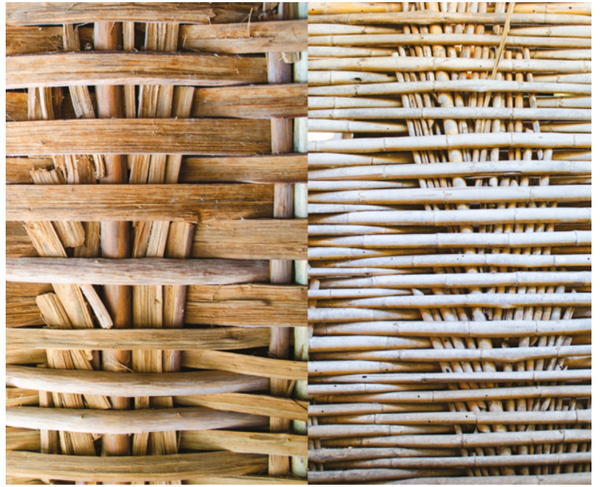
FIGURE 6. Comparison of two materials used for the framework of pajarete walls. Left: wall interwoven with blue mahoe; right: wall interwoven with open otate (cracked) (Photograph: Antonio Flores, 2018).
