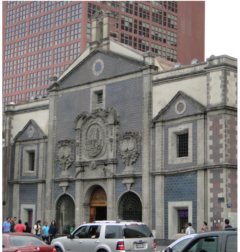
FIGURE 1. Corpus Christi convent main facade, Mexico City (Photograph: Ivan San Martín, December 2006).
