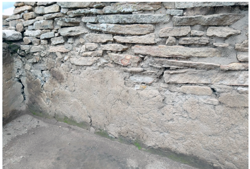
FIGURE 1. Remnants of a wall with earth-based flattening in the La Quemada archaeological zone, Zacatecas (Picture: Josué Israel Moreno Fraga, 2020; courtesy: Centro INAH Zacatecas).
