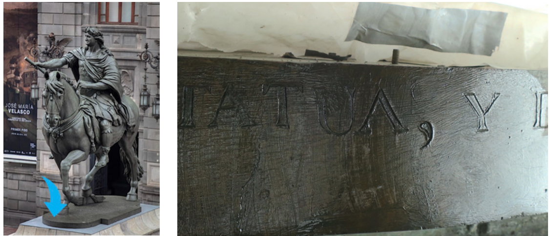
FIGURE 7. Location and detail of the screw at the front of the bronze base during the cleaning process. (Photograph: Francisco Kochen, taken from INAH, 2017. Right, Photograph: Jannen Contreras, 2017).
