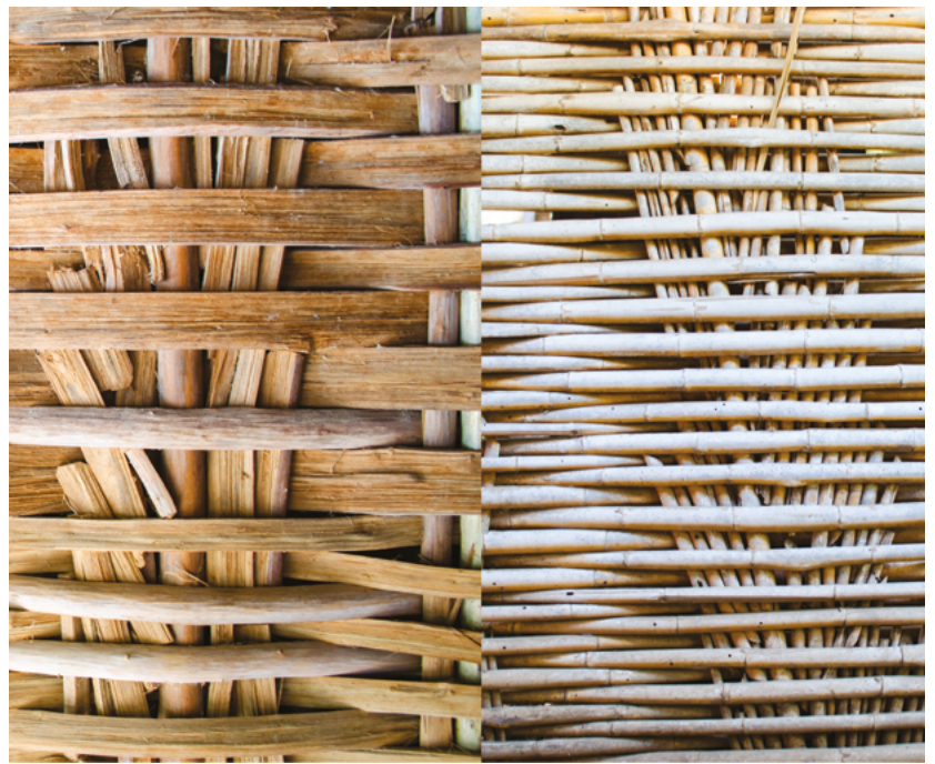
FIGURE 6. Comparison of two materials used for the framework of pajarete walls. Left: wall interwoven with blue mahoe; right: wall interwoven with open otate (cracked) (Photograph: Antonio Flores, 2018).
