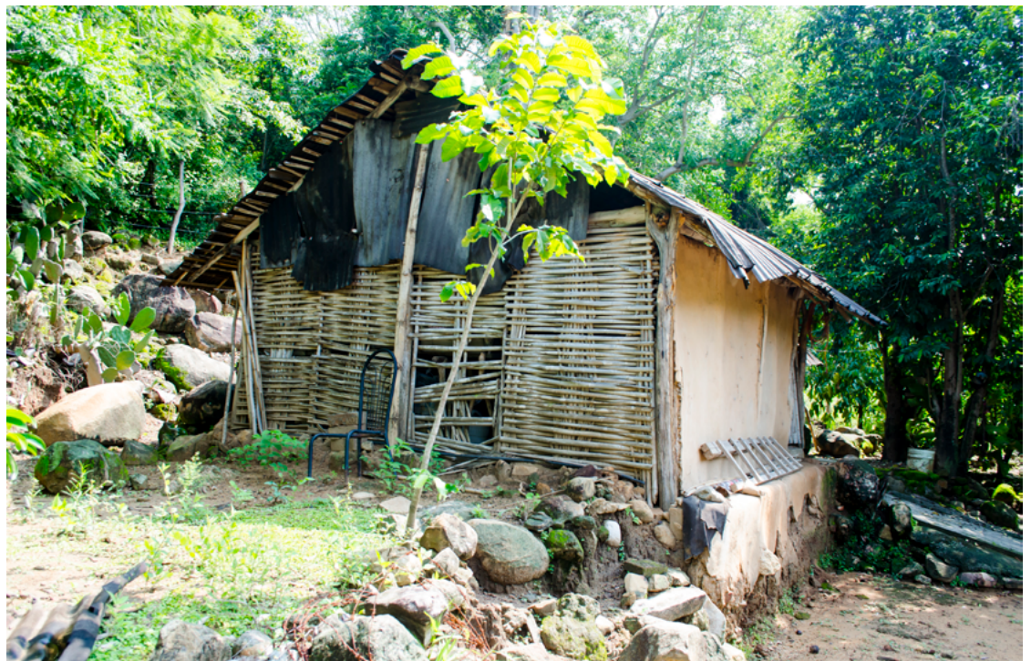
FIGURE 7. Pajarete house located in the community of Pueblo Nuevo displaying the walls of otate and the presence and absence of earth as a finish (Photo: Antonio Flores, 2016).
