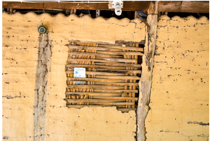
FIGURE 8. Detail of the type of window used in the pajarete houses in the Valley zone of the state of Colima (Photograph: Antonio Flores, 2016).
