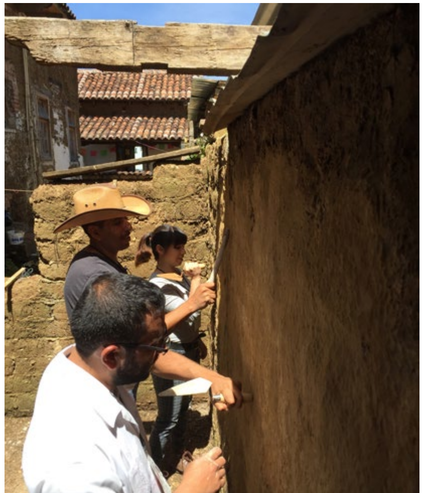
FIGURE 2. Restoration of an adobe wall during the workshop for conservators of the Centro INAH Chiapas. San Cristóbal de Las Casas, Mexico (Photograph: Luis Fernando Guerrero Baca, 2018).
