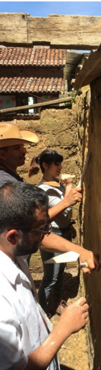
FIGURE 2. Restoration of an adobe wall during the workshop for conservators of the Centro INAH Chiapas. San Cristóbal de Las Casas, Mexico (Photograph: Luis Fernando Guerrero Baca, 2018).
