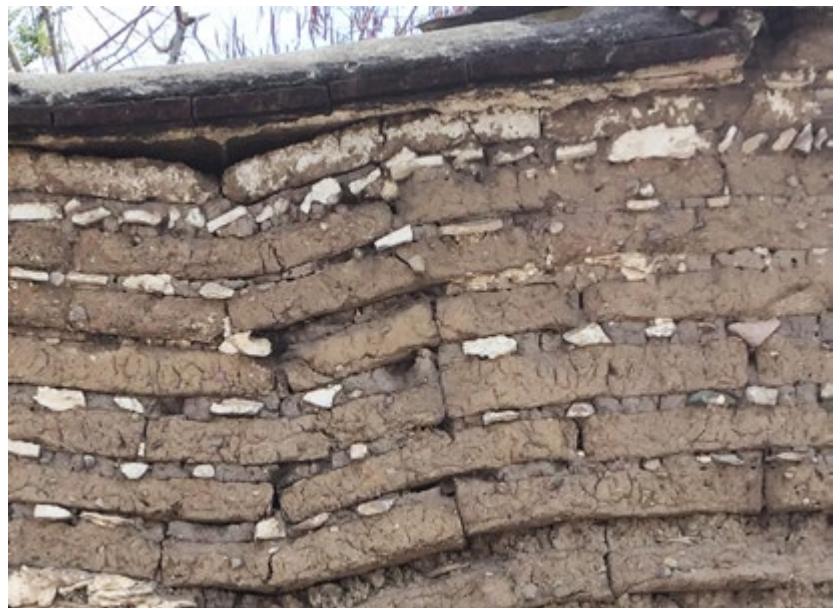
FIGURE 9. Adobe, unlike other masonry products, has the ability to deform within certain limits. Huehuatlán El Chico, Puebla, Mexico (Photograph: Luis Fernando Guerrero Baca, 2018).
