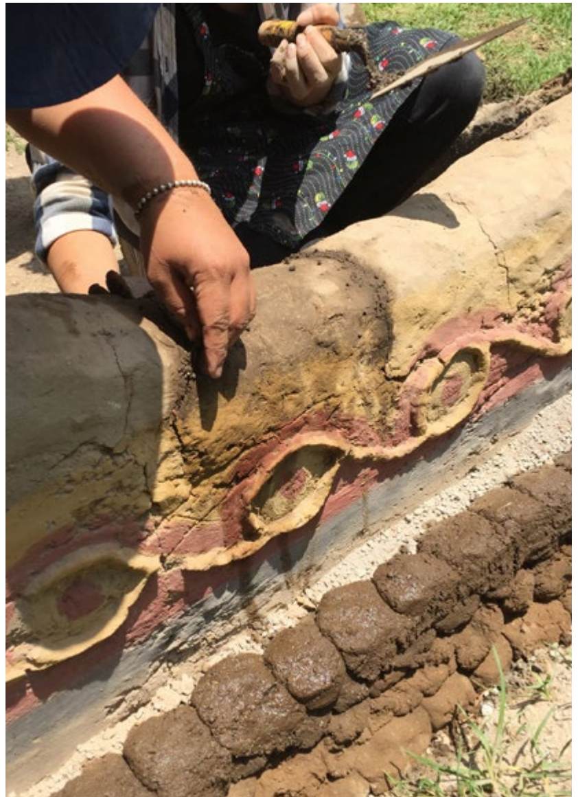
FIGURE 12. Practice of consolidation and re-burial using modeled soil in the classes of the Master's Degree in Conservation and Restoration of Built Heritage of the ENCRYM-INAH (Photograph: Luis Fernando Guerrero Baca, 2019)
