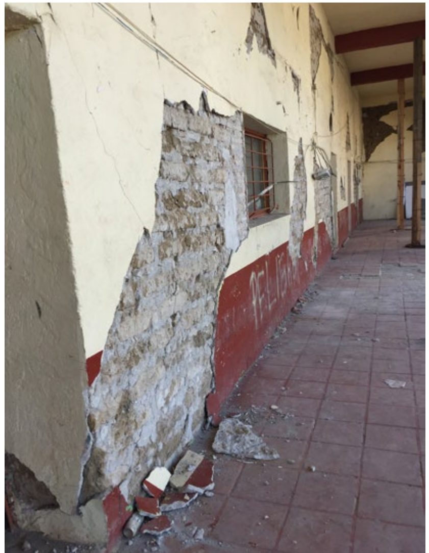
FIGURE 1. The cracks shown in the adobe walls covered with cement mortar were only superficial. Ayudantía Municipal de Hueyapan, Morelos, Mexico (Photograph: Luis Fernando Guerrero Baca, 2017).
