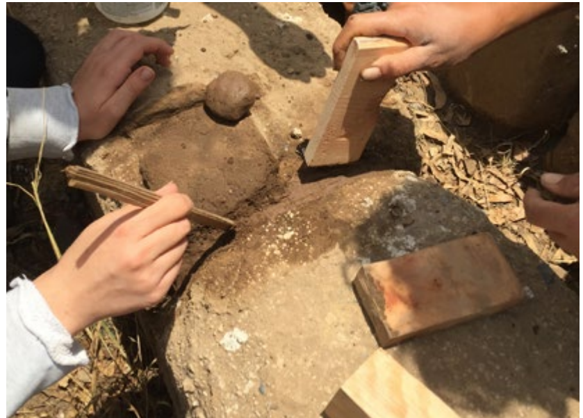
FIGURE 10. Refilling of cracks during a workshop of the Bioconstruction Immersion Program. San Isidro Project, Tlaxco, Tlaxcala, Mexico (Photograph: Luis Fernando Guerrero Baca, 2019).
