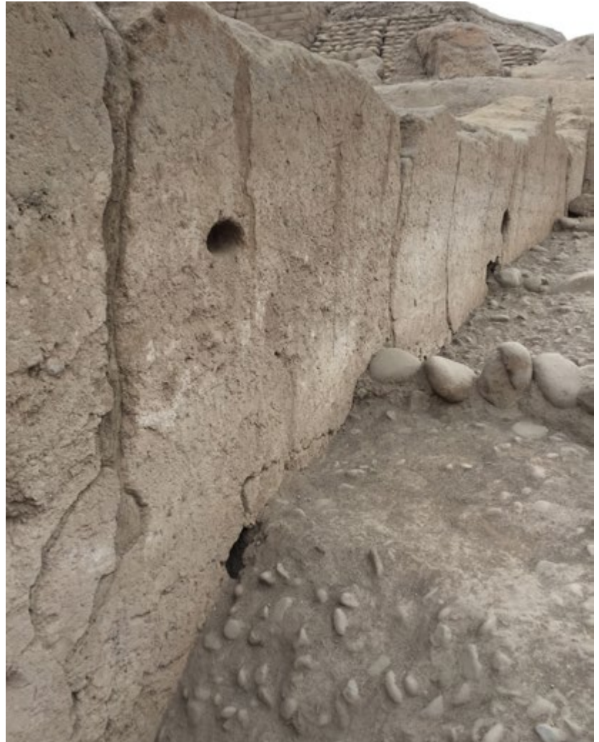
FIGURE 8. The archaeological walls of the Bellavista site in Lima, Peru, gave the false impression of having been built using the rammed earth technique, but their patterns of deterioration are evidence of the use of kneaded earth in a plastic state (Photograph: Luis Fernando Guerrero Baca, 2017).
