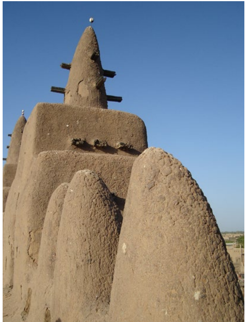
FIGURE 3. The use of clayey soils allows the production of less permeable finishes, but its cracking requires periodic maintenance. Crenellations of the Djenné Mosque, Mali (Photograph: Luis Fernando Guerrero Baca, 2008).
