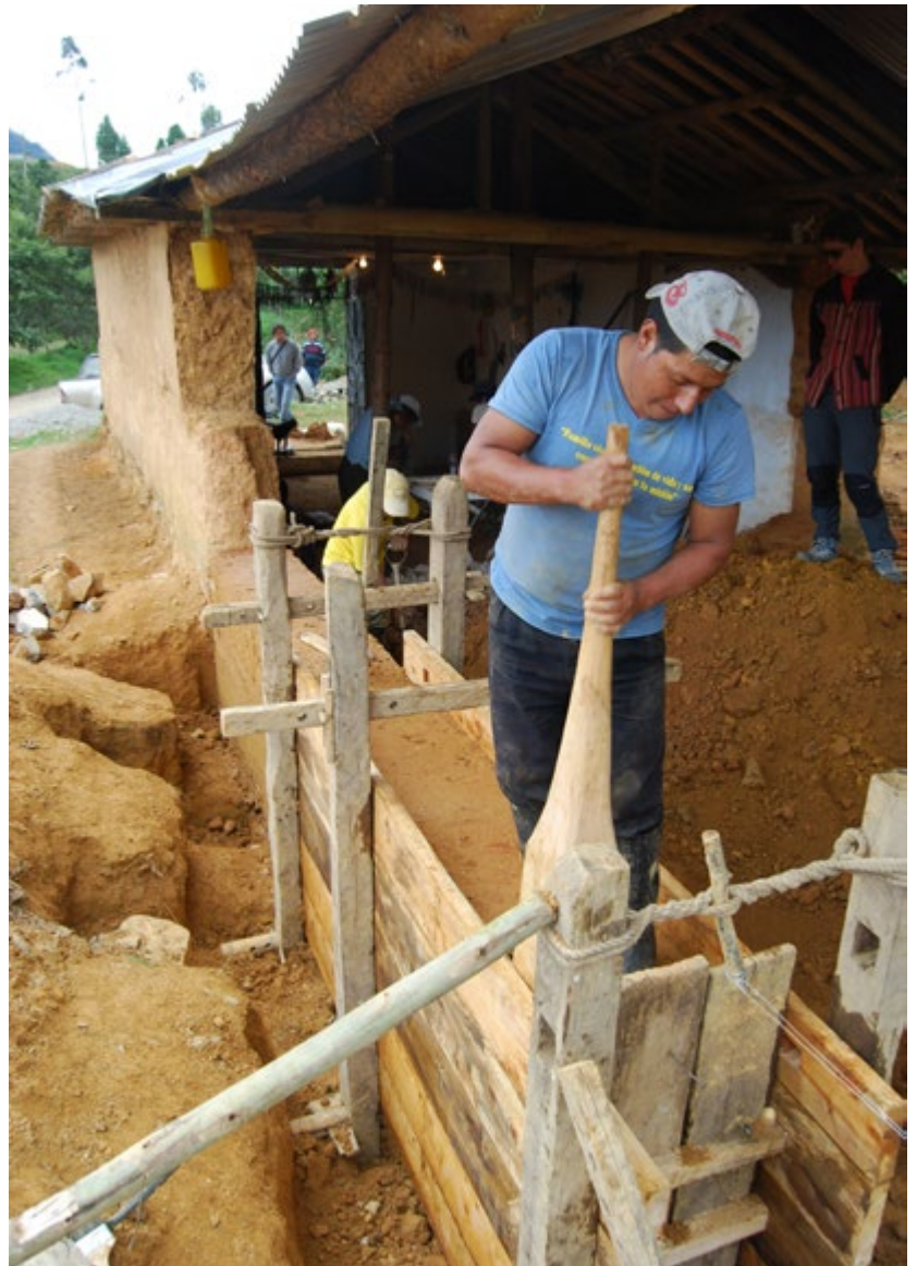
FIGURE 7. Restoration of a tapia heritage chapel in Chuquiribamba, Ecuador (Photograph: Luis Fernando Guerrero Baca, 2014)
